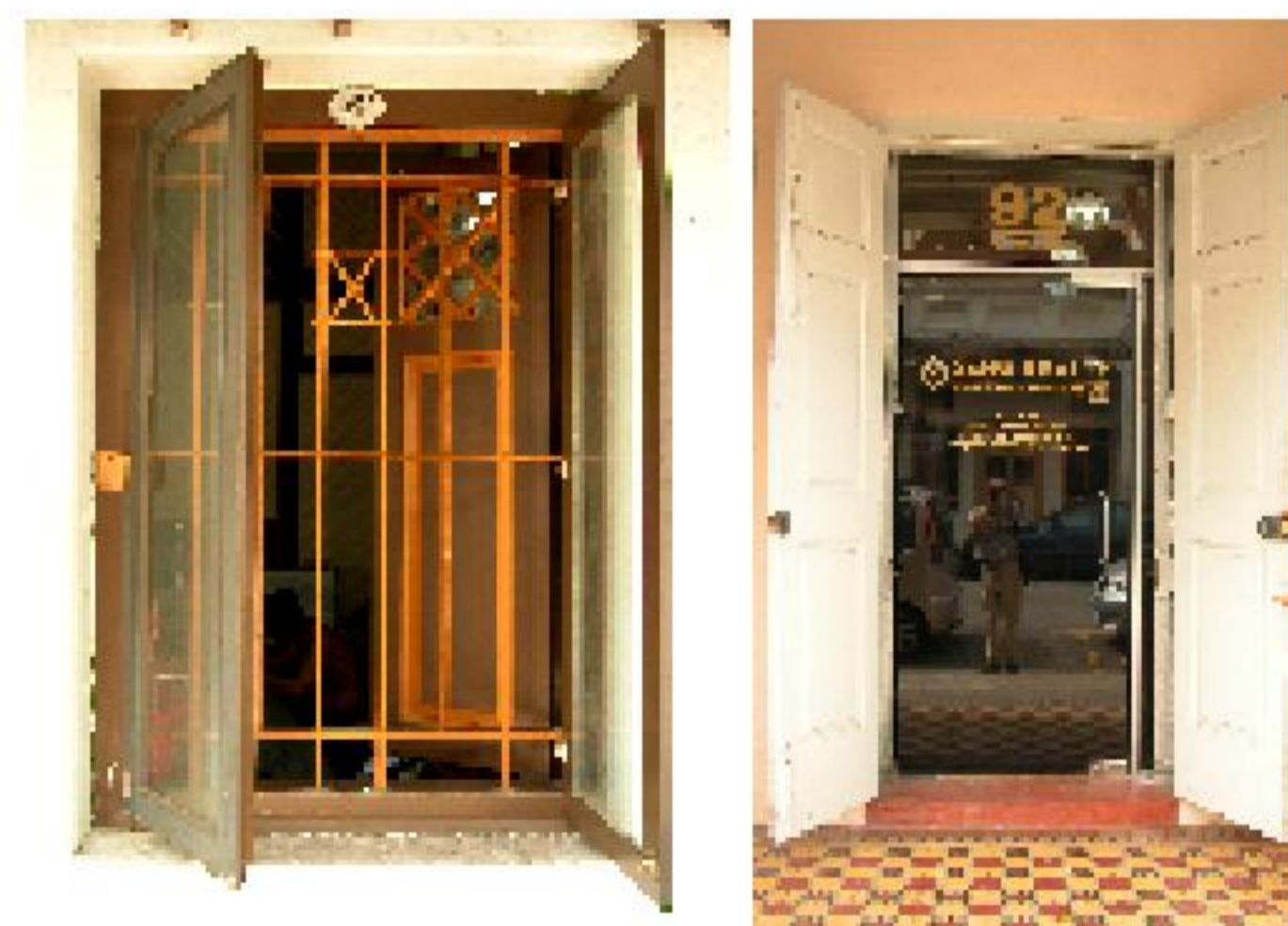
Incorporating glass over traditional door and window
